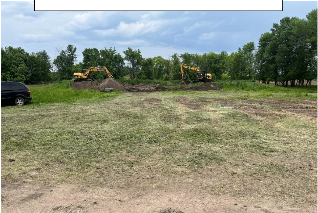
Earthwork completed by Didier Excavating.
